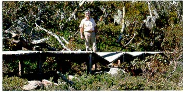
Tracks such as the Charlotte's Pass walkway require annual maintenance by the National Parks and Wildlife Service. The weight of snow on the raised walkways causes them to bend or break under pressure.
